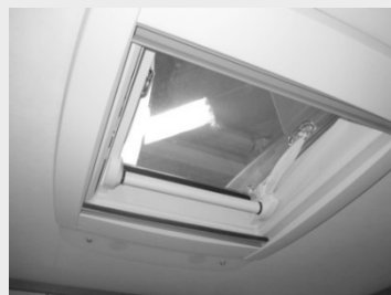
Afb. 35: Dakluik 400x400 mm VisionStar 700x500 mm
